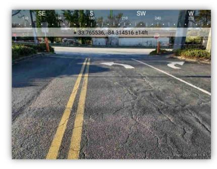
East Lake Station - alligator cracking and rutting in pavement.
