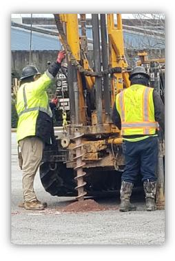
Kensington Station – drill rig performing soil test borings.
